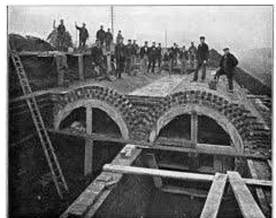
NORTHERN OUTFALL SEWER IN COURSE OF CONSTRUCTION. 1860-67.
